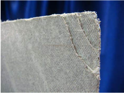
Asbestos Cement Panel
