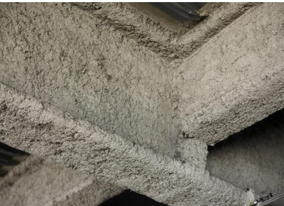
Asbestos Spray –applied
